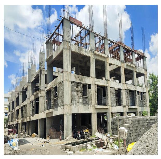
**Block C1: Terrace Floor** level slab concrete 100% completed. Parapet Column concrete 100% completed. Block work in Tenth floor 70% completed.
