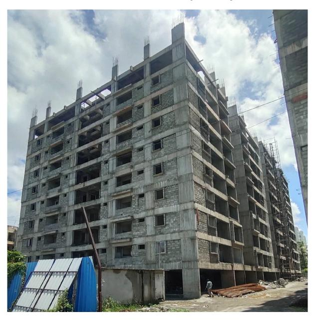
Community Hall: Parapet Column concrete casting 100% completed. External Plastering in West side elevation 95% completed, South side elevation 85% completed & North side elevation 45%, East side elevation 50% completed.
