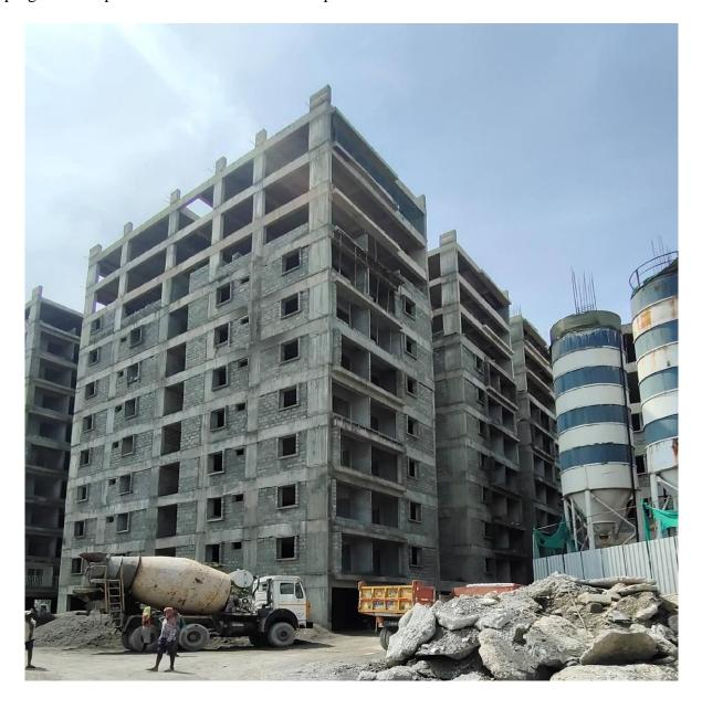
**Block C3:** Seventh Floor level slab Concrete casting 100% completed. Shuttering works for 1<sup>st</sup> half of Eighth floor level slab 20% completed and balance works on progress.
