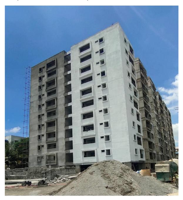
**Block B2:** Third Floor Level slab concrete casting 100% completed. Shuttering works for 1<sup>st</sup> half of Fourth floor level slab 15% completed.
