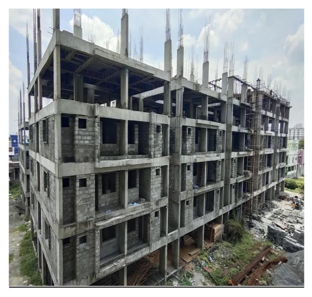
**Block A2:** Fifth Floor Level slab Concrete  $1^{st}$  half casting 100% completed Shuttering & Barbending  $2^{nd}$  half of Fifth floor level slab on progress.
