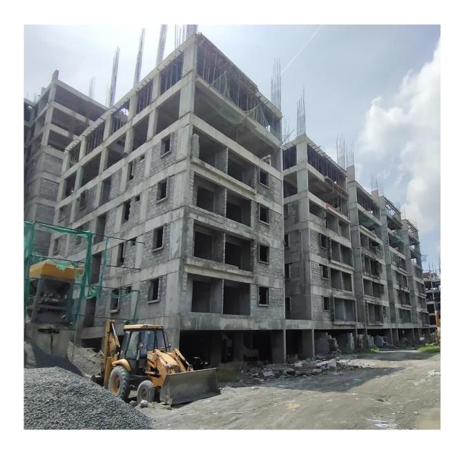
**Block D1:** Eighth Floor level slab Concrete casting 100% completed. Shuttering works for 1<sup>st</sup> half of Ninth floor level slab 95% completed.
