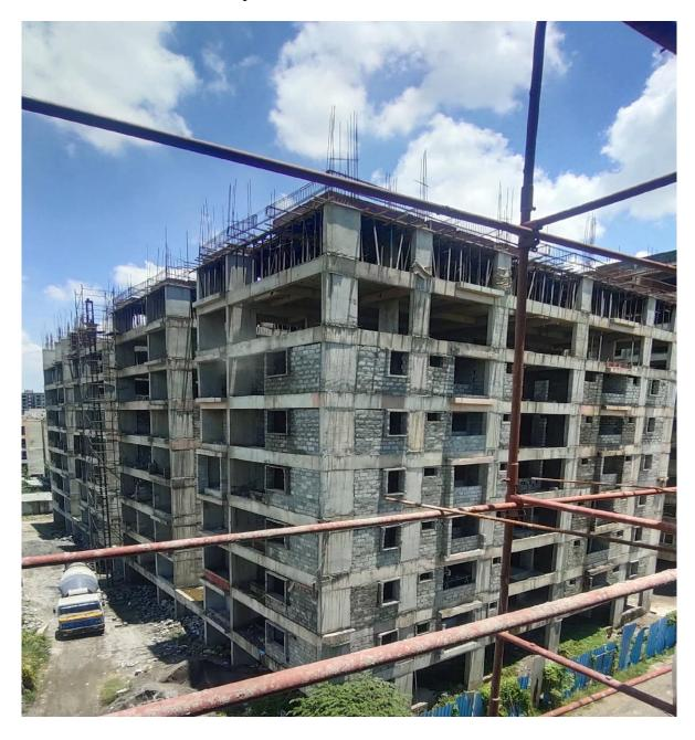
**Block D2:** Terrace Parapet Columns concrete 100% completed. External Plastering work in West side elevation 25% completed.
